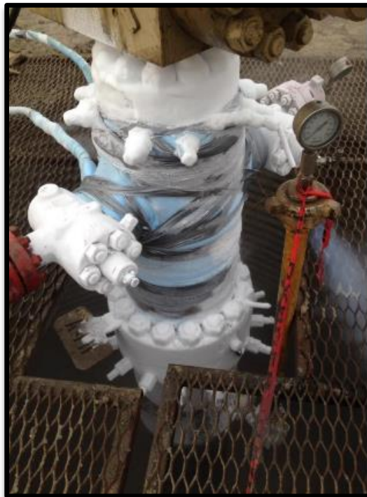
Figure 6: Cryogenic Freeze operation
