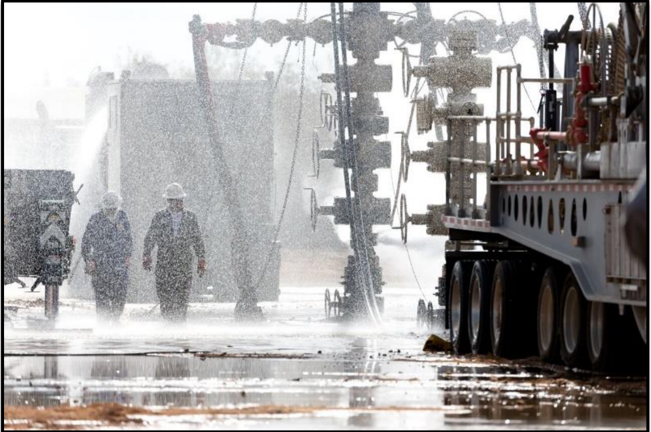
Figure 11: Fire pumps providing deluge for WC Ops
