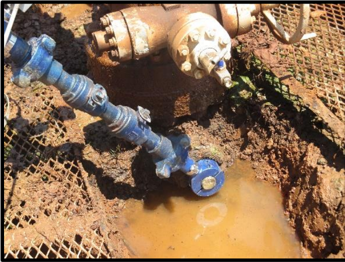
Figure 16 - Bull Plug Saddle Clamp
