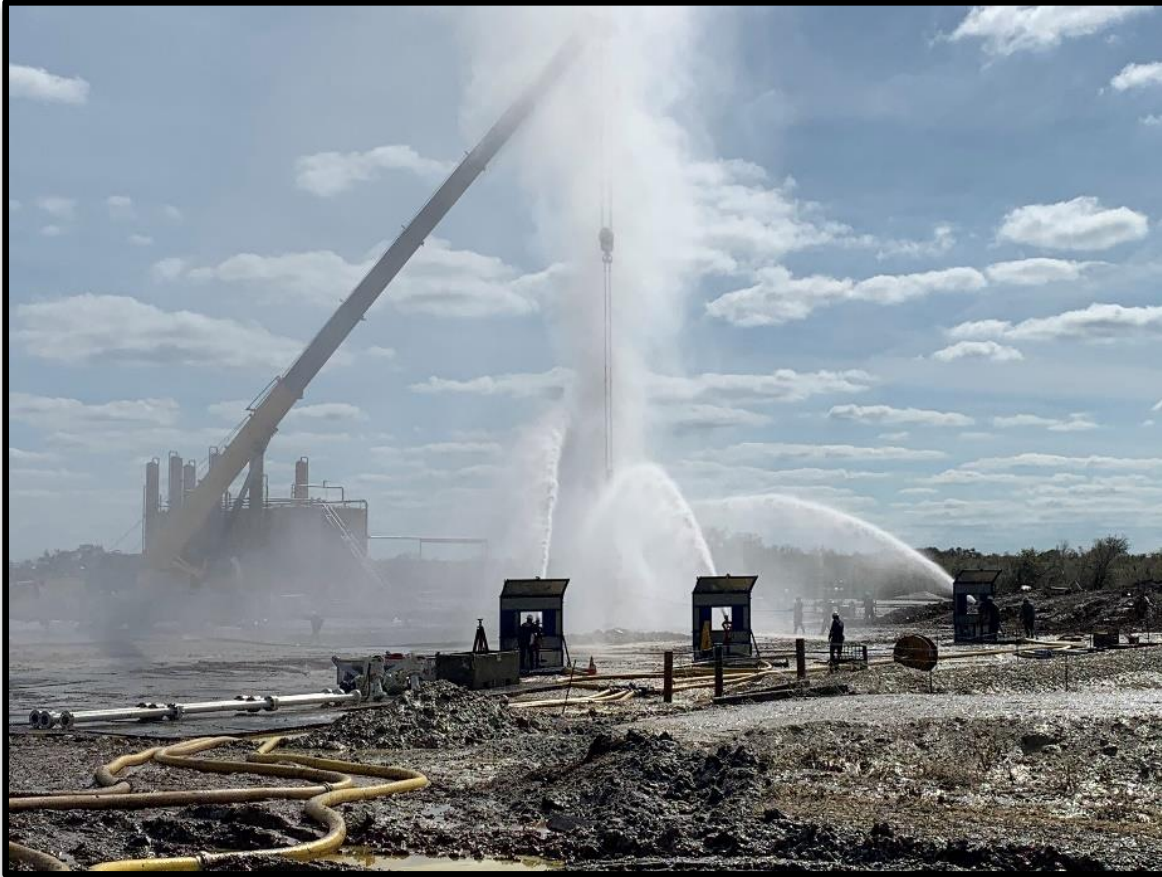
Figure 4: Capping with 11" 10M Capping Stack
