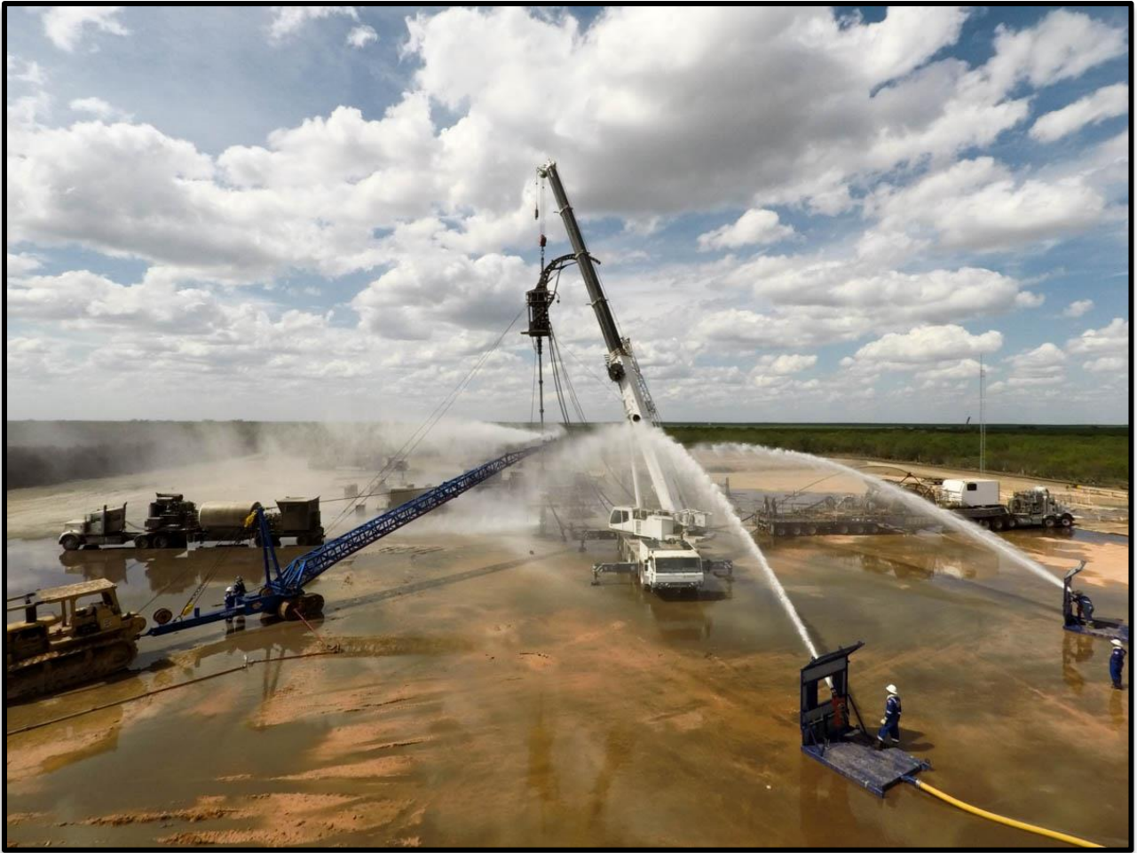
Figure 12: Providing suppression during an AJC cut
