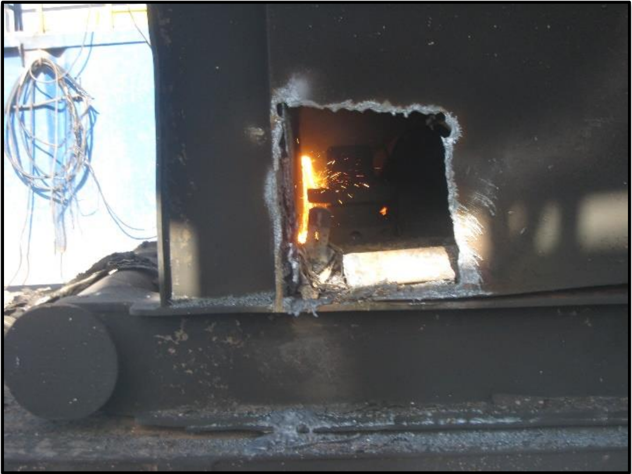
Figure 10: Cuts made by an Exothermic Torch
