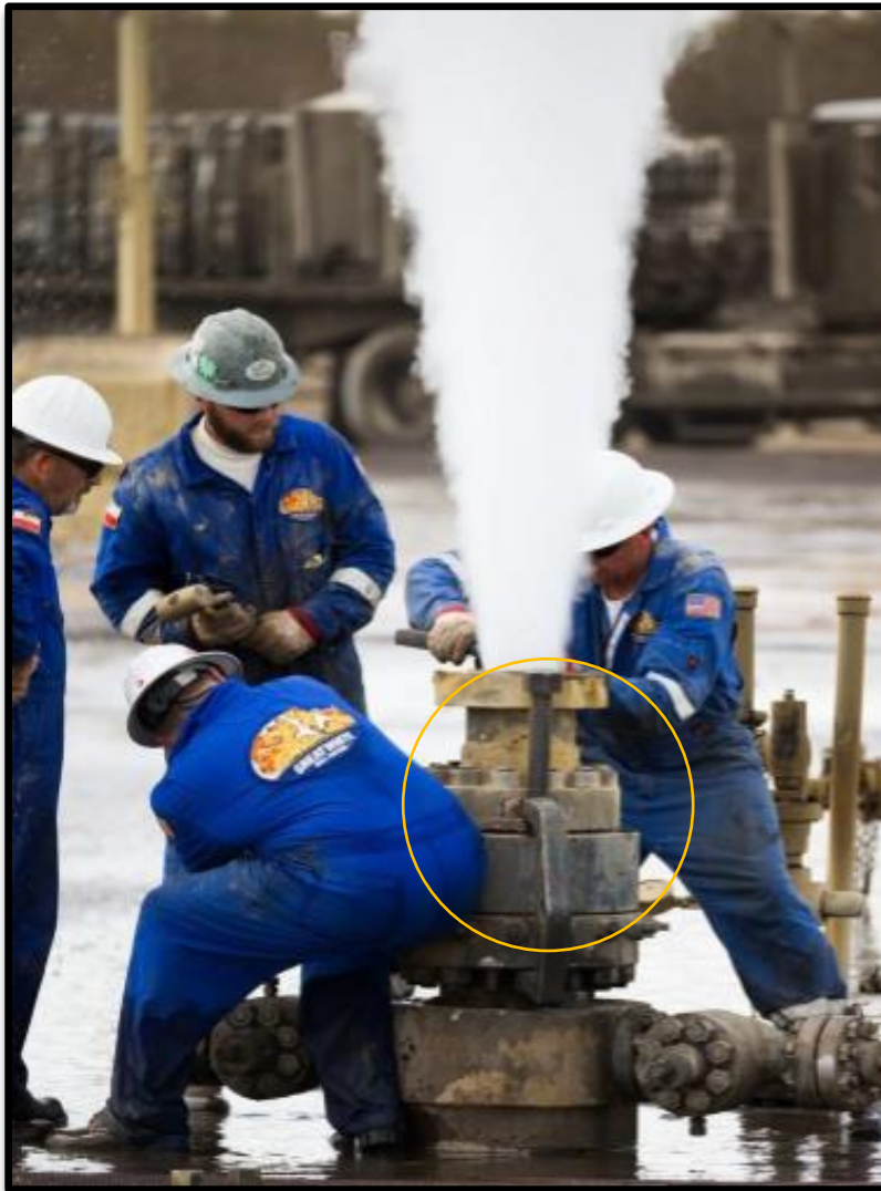
Figure 3: C Clamp for head removal
