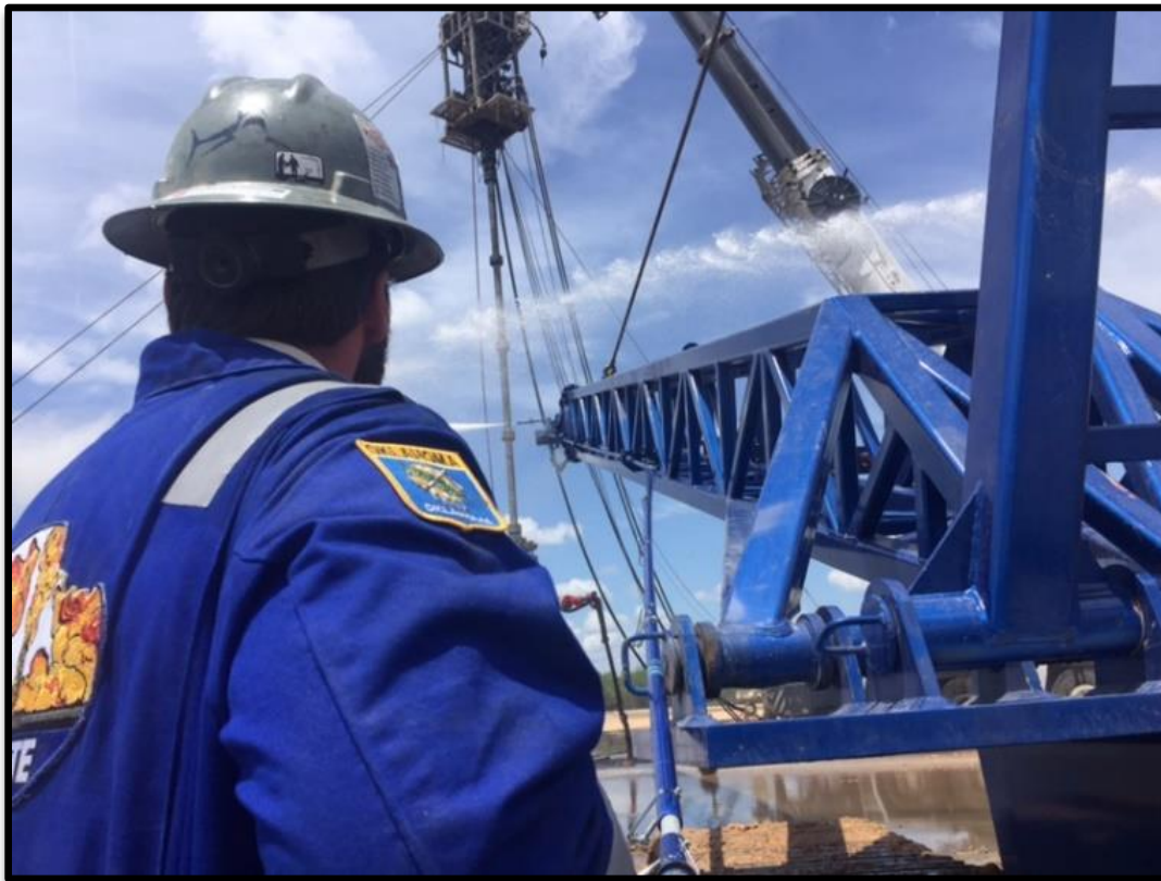
Figure 1 : AJC making a cut on CT Lubricator
